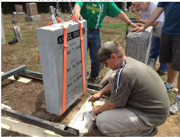
James Long placing the new Asael Smith headstone encasing the old one
