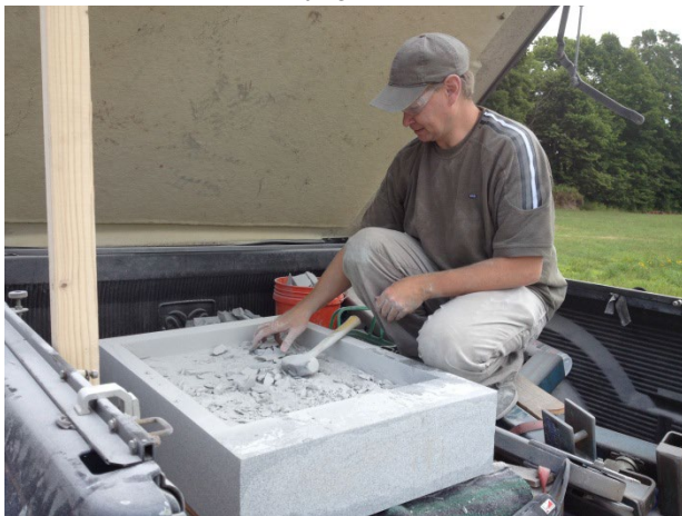
James Long taking out the extra stone to place the old stone
