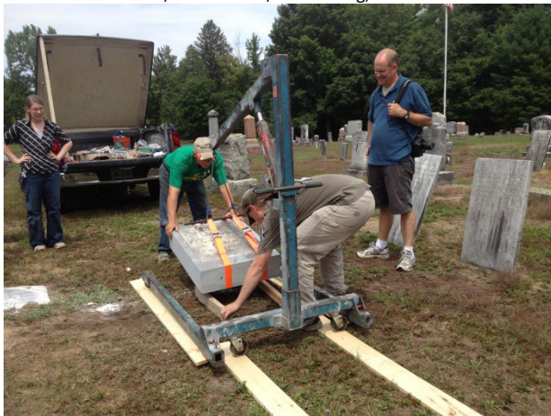
Meghan Long, Dick Hann, James Long, and J.C. Sorensen prepare the ground which was very soft with wood to keep the hoist from sinking while moving the heavy stone
