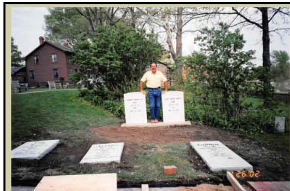
A Work in Progress
